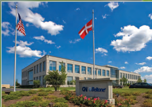
Belton headquarters – a 50,000-square-foot Catellus build-to-suit development at Prairie Glen Corporate Campus
