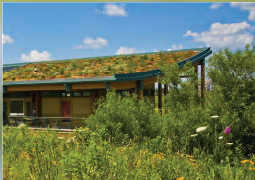
Catellus was a key contributor to the Evelyn Pease Tyner Interpretive Center at Air Station Prairie – certified LEED® Platinum by the U.S. Green Building Council
